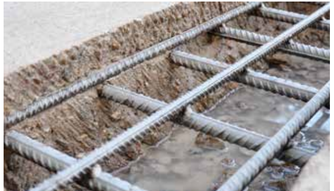
Hydromilling - Concrete removal using high pressure, ~2000-3000bar.
