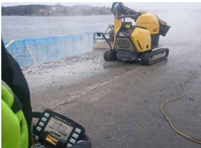
The robot is remotely operated which makes the process efficient and safe.
