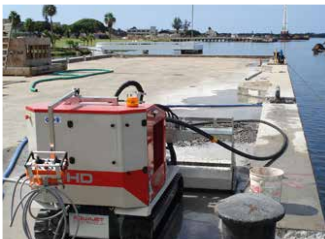
An early version of a hydrodemolition robot removing concrete at Pearl Harbour.
