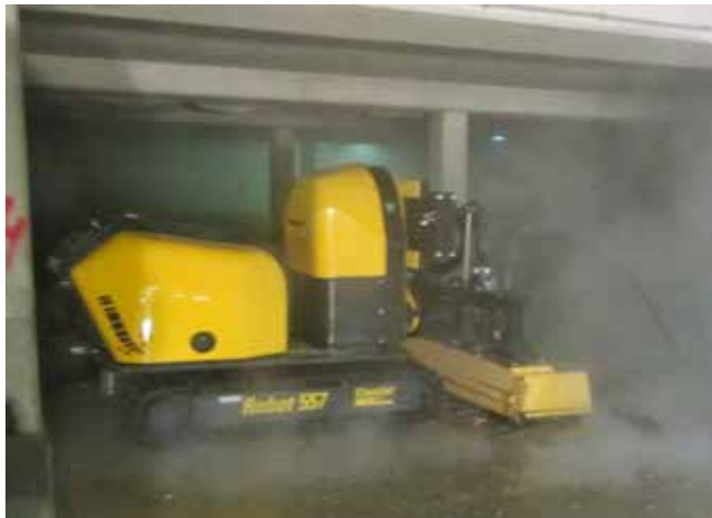
Robot removing the deteriorated concrete on a slab in a car parking.
