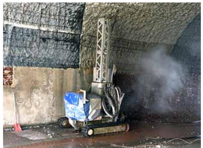
The Robot is removing the vertical surface along the tunnel.
