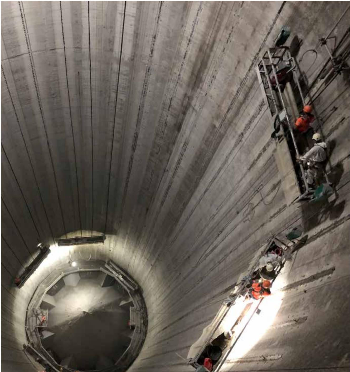
Internal restoration of a Silo in Spain.
