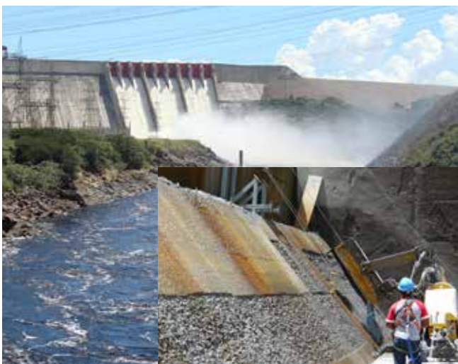
The spillways were refurbished on the Gori dam in Venezuela. The equipment was operated from a movable platform.
