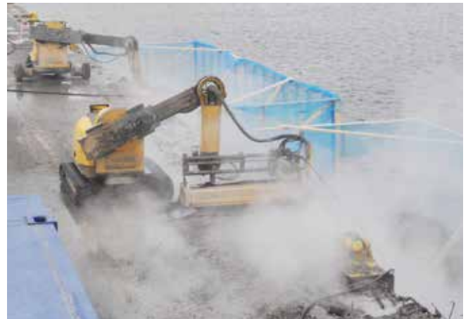
Viking terminal in Stockholm being refurbished. One robot is removing the horizontal part and the other the vertical part of the quay.
