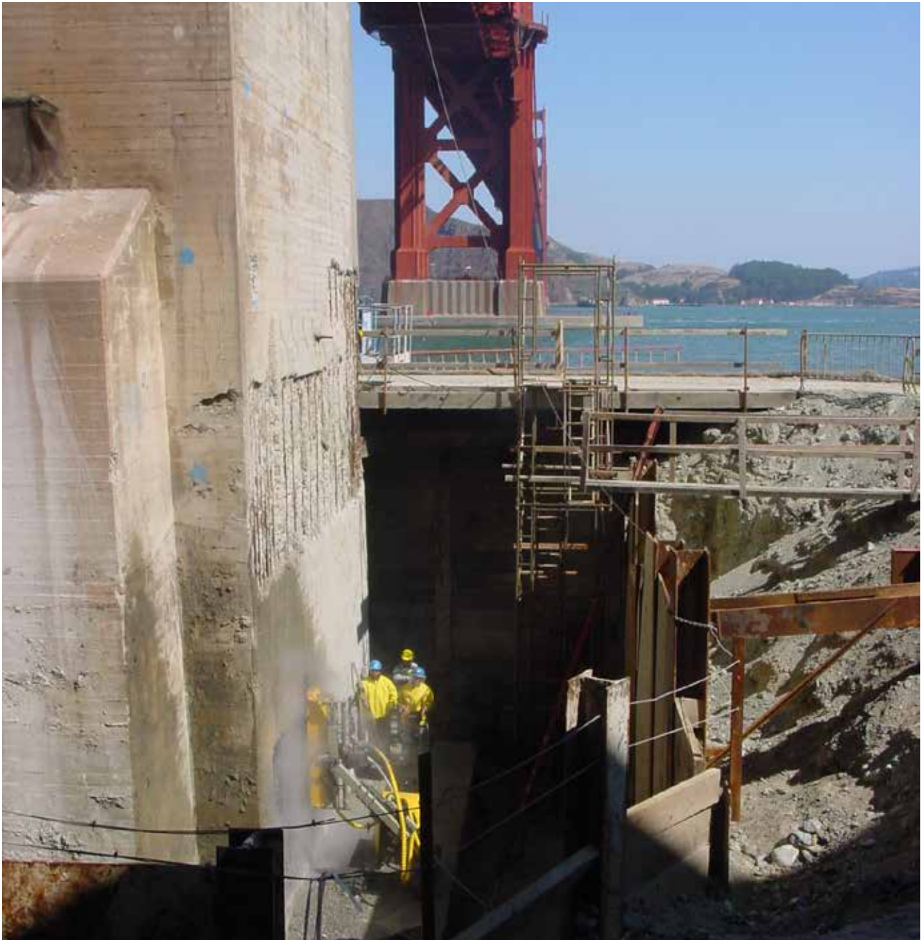
Gold Gate Bridge in San Francisco, CA, USA Preparation of the concrete surface to enclose the entire pillar with a steel structure to strengthen the pillar as a safety precaution against the possibility of earthquakes that can occur in the region.
