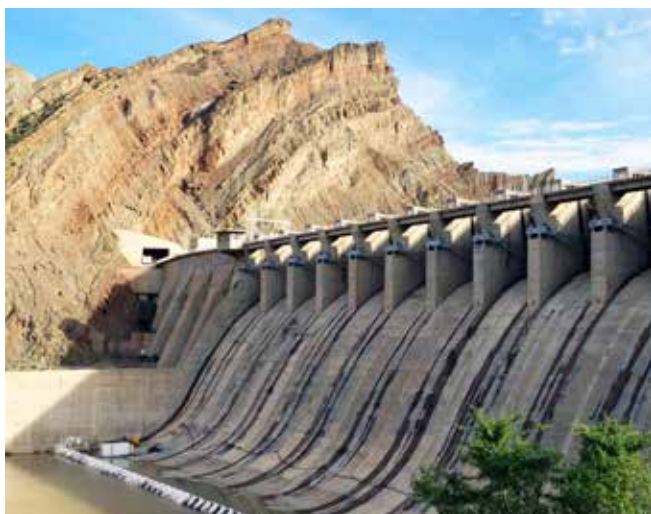
Deteriorated concrete being removed by robot at Minab dam in Iran.
