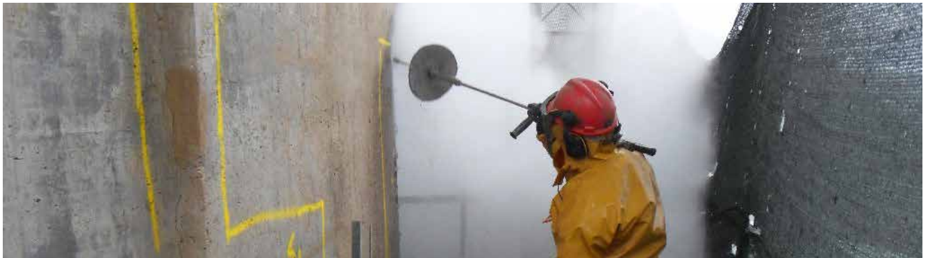
Hand lance operation is sometimes needed in confined areas where it is difficult to use a robot or the concrete quantity to be removed is limited.
