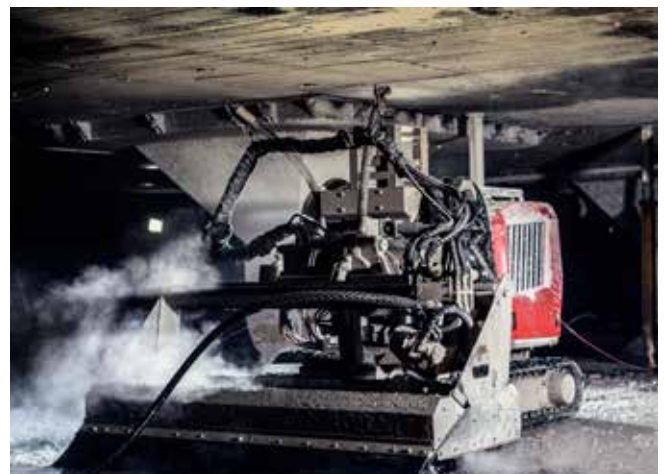
Robot in operation, the picture shows the cutting head moving from side to side.
