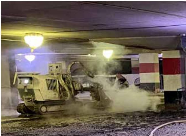
Restoration of a car parking deck.
