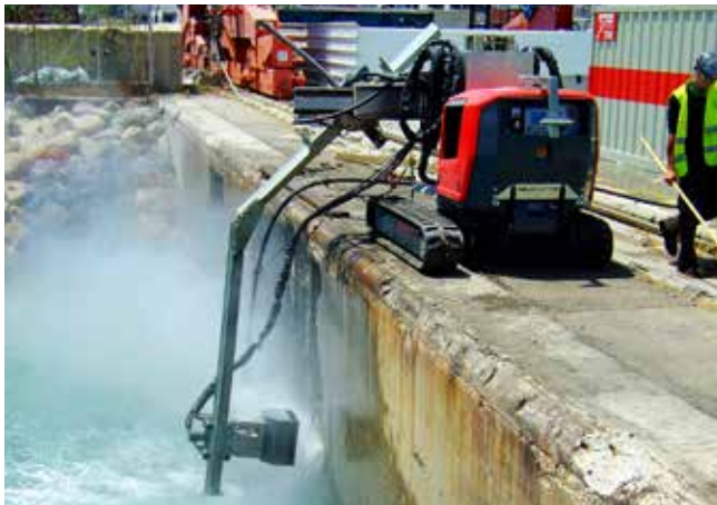
Deteriorated concrete is being removed at the Port of Haifa, Israel.
