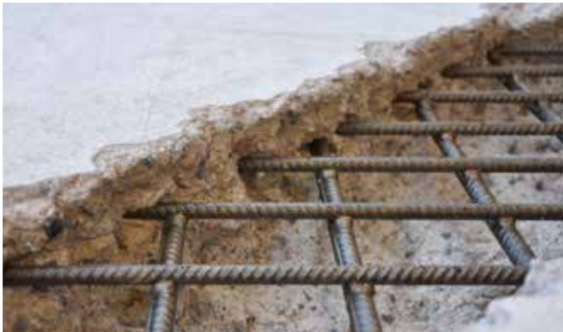
Hydrodemolition - Concrete removal using high pressure, ~1000-1600bar.
