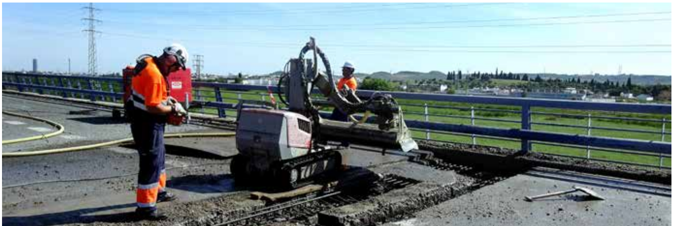
Bridge joint being removed, Rebars remain intact, so it is easy to replace the joint.
