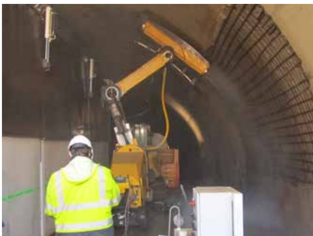
Robot is removing concrete, operating from a train wagon so the equipment can be moved fast in and out of the tunnel.
